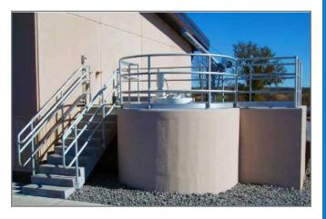
Constructed from 6005-T5 SCH 40 aluminum alloy pipe with SCH 80 posts and spaced not more than 5' on center. BMC railing is unique in the industry due to the use of 304 stainless steel flanges. Stronger than aluminum and noncorrosive, they are polished to a #4 brushed finish to provide an attractive appearance.
